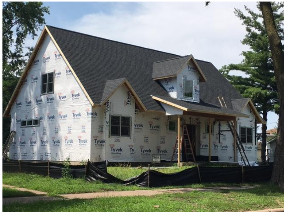
A Promise home being built on 5th Avenue.
