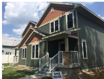
Twindo: 807-811 6th Street
